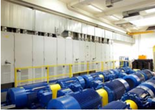
Endurance run test bays up to 270 kW in Siemens Ruhstorf factory
